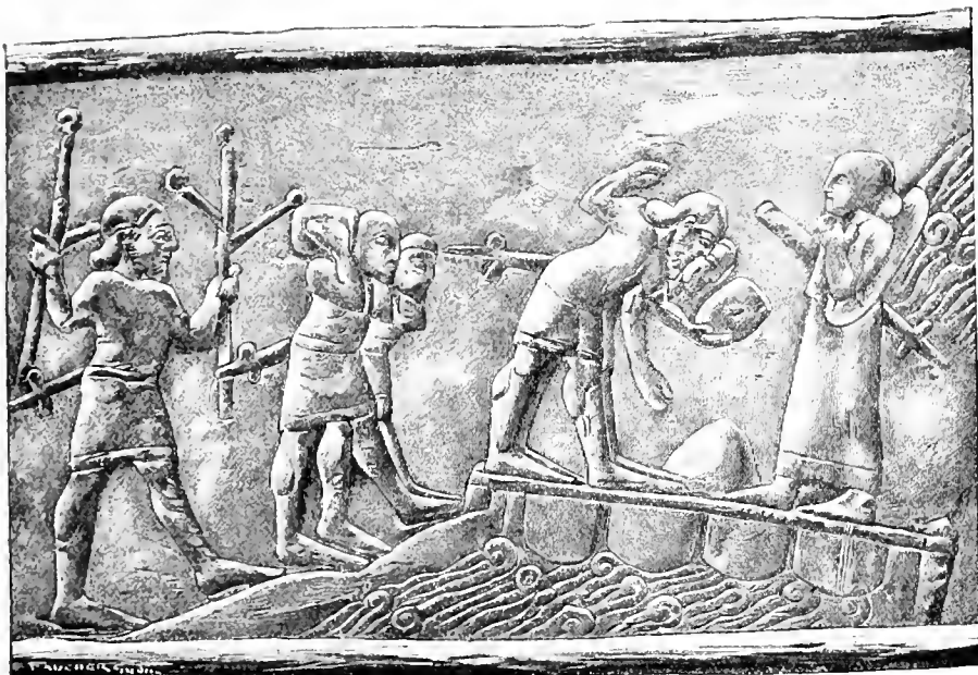
MAKING A BRIDGE FOR THE PASSAGE OF THE CHARIOTS. 1
